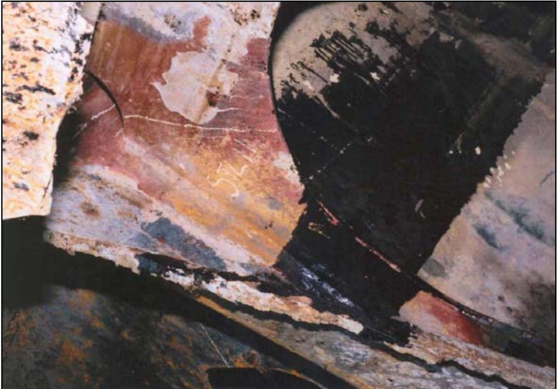
Transverse floor and longitudinal girder number 3 at 6050mm off centre line (including fillet weld connection) inside sea chest, frame number 84 starboard side prior to removal from the vessel
